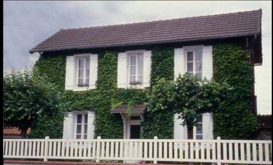
The “Maison Feuillette” in France, a timber frame in filled with straw bales which were then rendered, has been built in 1921 near Paris<sup>1</sup> and is still in use to this day.
